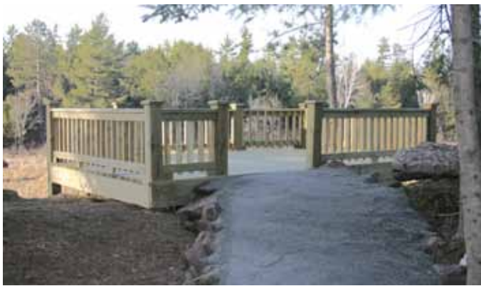
New Universal Design Trail Lookout – railing to be completed in spring
